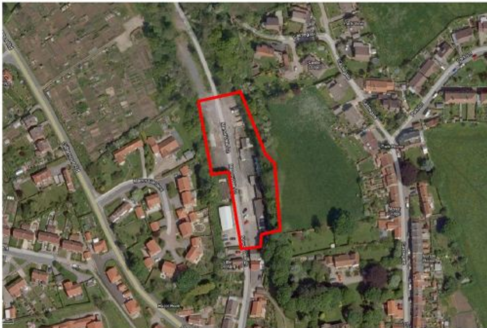
AERIAL VIEW OF EXISTING SITE
